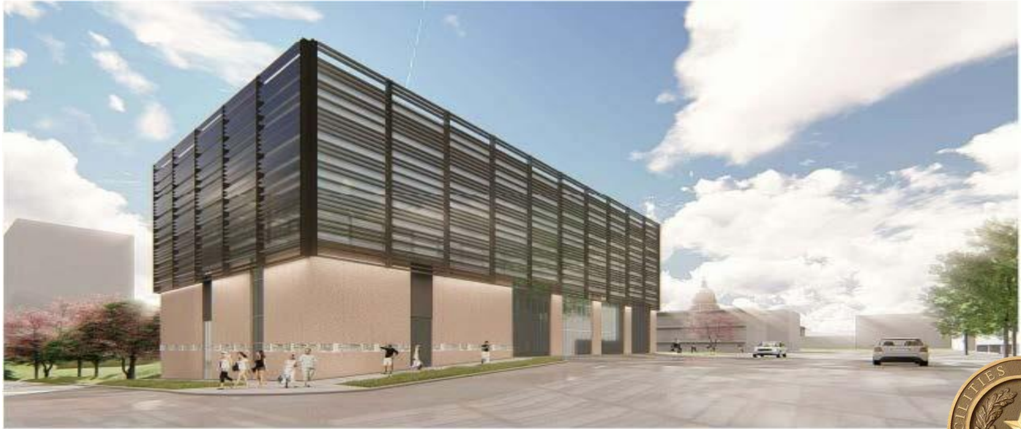
Central Utility Plant
